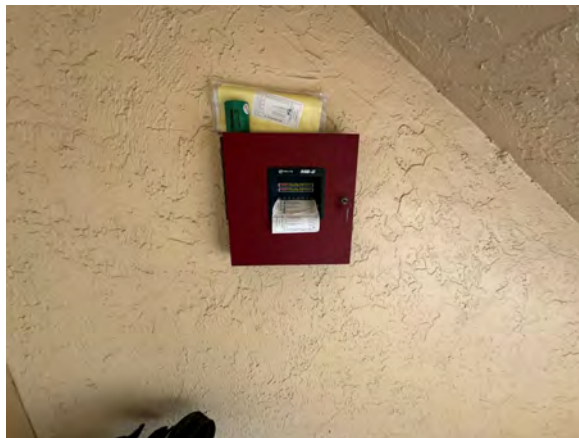
GENERAL VIEW OF TYPICAL FIRE ALARM CONTROL PANEL
